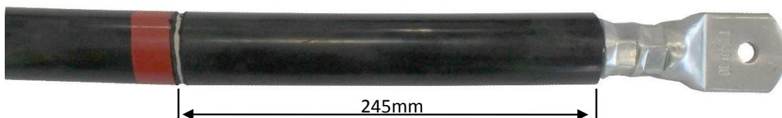
4. Remove tape used for marking distance. Use a heat gun and a box cutter to remove the 230mm of black outer semi-conductive sheath from cable (white insulation to remain).
