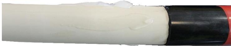
7. Place the cold shrink tube over the cable so that the end of the tube lines up with the tape used to mark 50mm. Ensure that the tube is placed in the correct direction (the end which has a wider diameter should be furthest from the lug) and that the plastic release “pull-strip” is fed through the tube and hanging out next to the lug. Hold in place and pull the plastic strip to release. The cold shrink tube should shrink tight against cable.
