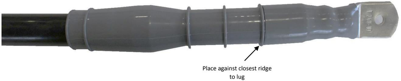
10. Place 0.5mm neon cable against the left of the first ridge and tape down. Moving from right to left, make 8 spirals and completely cover with tape to firmly hold in place.
