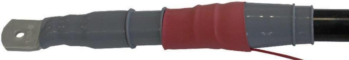
12. Strip back earth wire approximately 400mm to allow 3 complete rotations around the cable. Twist off and secure around cable and then tape down with earth tape.
