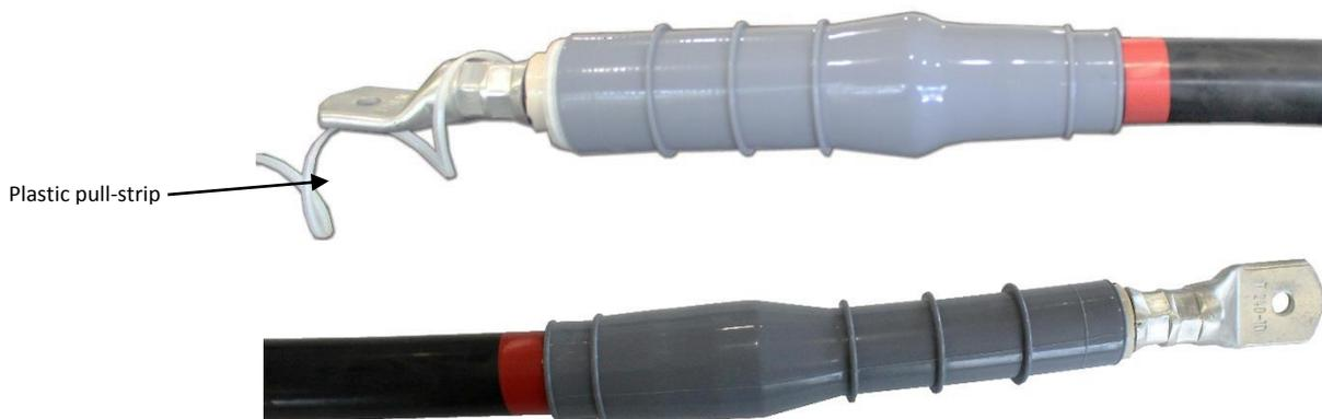
8. Add self adhesive tape (from kit – wrapped in yellow paper) to the end where the insulation and lug meets.
